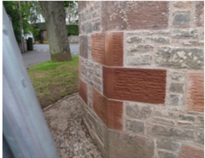
Masonry is designed to be repaired piecemeal: here, failed stones are cut out at Bowden Pant (1861, Category C(S)) by a mason from McIntyre Masonry. The completed repairs, above right, will blend in harmoniously over time.
