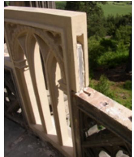
*Rebuilding the balustrade at Brizlee Tower included adding stainless steel posts to support and reinforce the balustrade to make it safe.*
