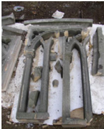
*Many of the balustrade panels at Brizlee Tower, Northumberland (1781, Grade I) were beyond recovery due to rusting of the original iron pins and cramps and had to be completely re-carved in matching sandstone. Stainless steel and bronze cramps and pins were substituted in the repair work.*
