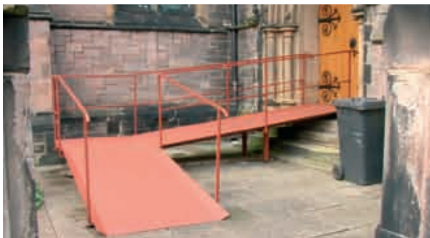
An ugly temporary ramp
