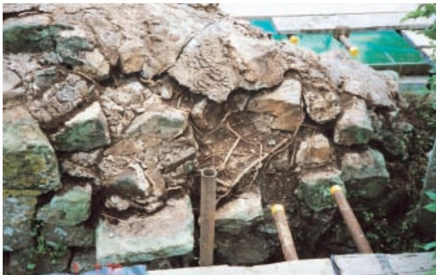
*Hard cement capping after clearance, showing extensive root penetration into the wall head.*
