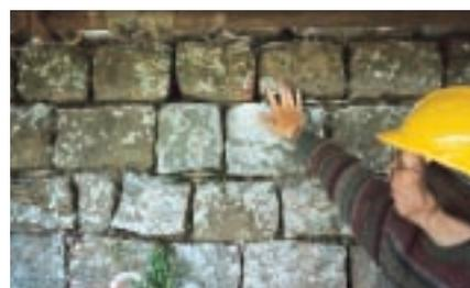
*Cavities used as bat roosts can be identified and marked with coloured crayons to ensure that they are preserved when repointing is carried out.*
