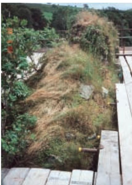
*Roses and other woody vegetation have led to fracturing, disintegration and progressive collapse of the wall head.*
