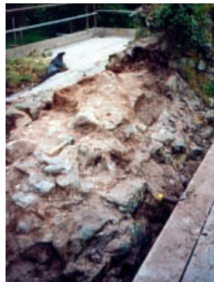
*Grass and non-woody vegetation removed from wall heads can be retained on plastic sheeting with hydroponic gel, and watered regularly.*
