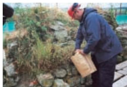
*To ensure that the soft top retains its authentic character, seeds are collected before stripping the 'natural' soft top and consolidating the masonry.*
