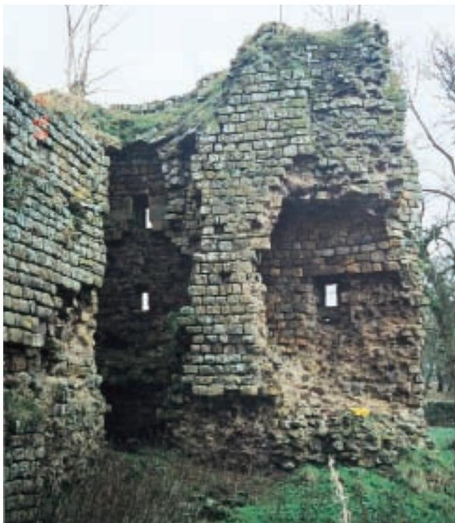
*Inadequately supported massive masonry which requires the introduction of new supports.*
